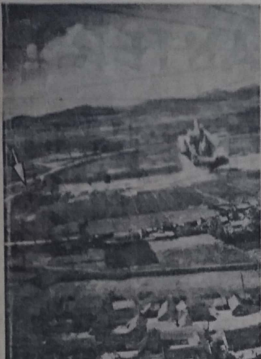
JAPS BRIDGES KEEP 'FALLING DOWN' —Last February medium members of the Fourteenth Air Force knocked-out the railroad bridge, north, left, across the long Chi river in French Indo-China, immediately north of Thanh Hoa. The Japs constructed a by-pass bridge, center, to handle freight across the river which was completed late in April. On May 10, Flying Tiger Mitchells staged a raid on the new bridge. The result, pictured above, a direct hit on the bridge which knocked-out 40-feet and rendered it useless. Other bombs tore the trestle and approaches to the bridge. The rail-road is the main communication and supply line for the Japs between Hanoi and Tourane.
