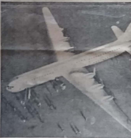
WORLD'S LARGEST transport, this Vultee plane will carry 204 passengers and 15,000 pounds of baggage, mail and express. Streamlined slipper is 13 times the size of standard commercial aircraft, and is powered by six engines which produce power equal to that of 353 automobiles. Plane is 182 feet long.
