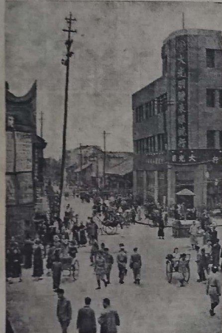
SOUTH END OF SCHUEN SHE ROAD at the inter-section of Chung Foo Street, looking west on Chung Foo.
