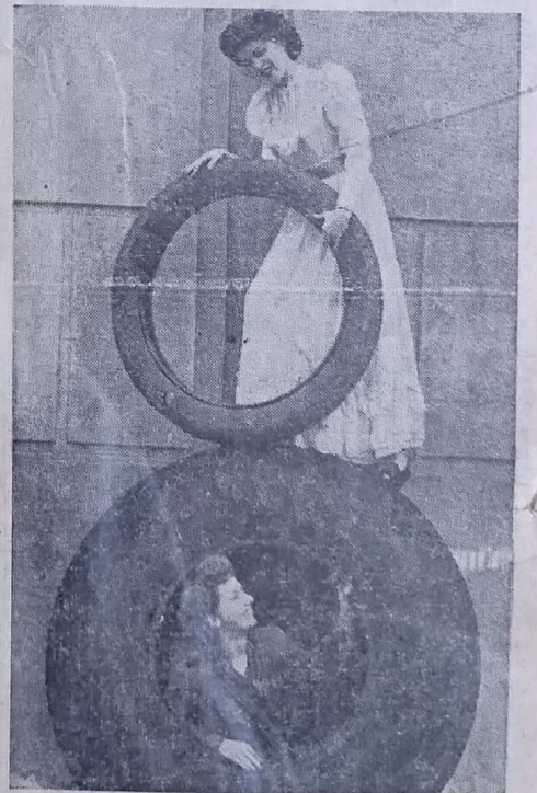
THE OLD AND THE NEW —Displacing 1915 model high-pressure tire, Luella Hammond (top) poses in old-time costume. In contrast is huge bomber tire (below) that frames Joyce Forbes. New type tire is made with nylon cord and metal cups, and weighs 276 pounds.
